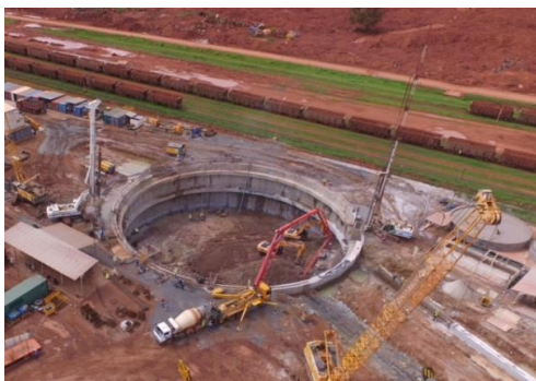
Figure 2. Crusher pit excavation.
