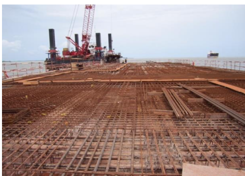
Figure 4. Mineral quay deck construction.
