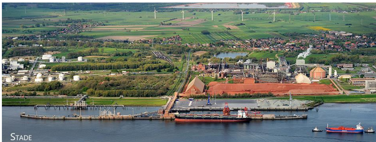
Figure 1. Aerial view of AOS.
